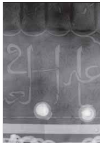
Figure 4. Two of the rivets and a cluster of fissures.
